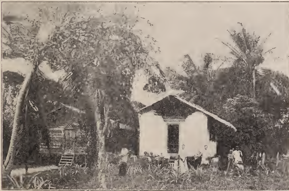
SCHOOL ON CORISCO ISLAND, WEST AFRICA
